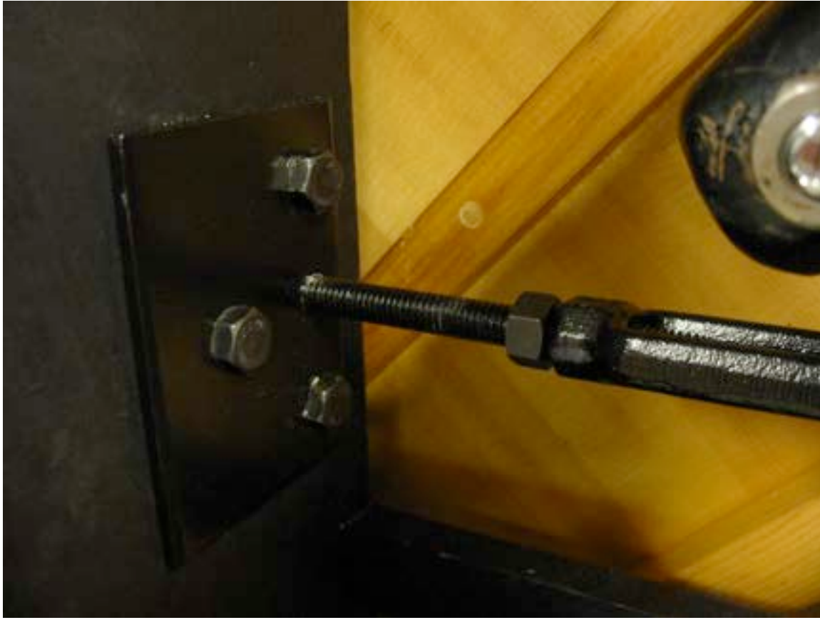
Photo 7 Final installation of the Belly Plate lag screws
