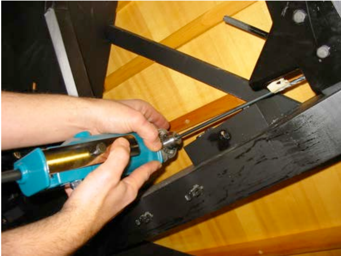
Photo 5 Utilizing an extended length drill bit for the tight spots
