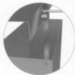
FIGURE 12 Hangers go on the outside of the baffle
